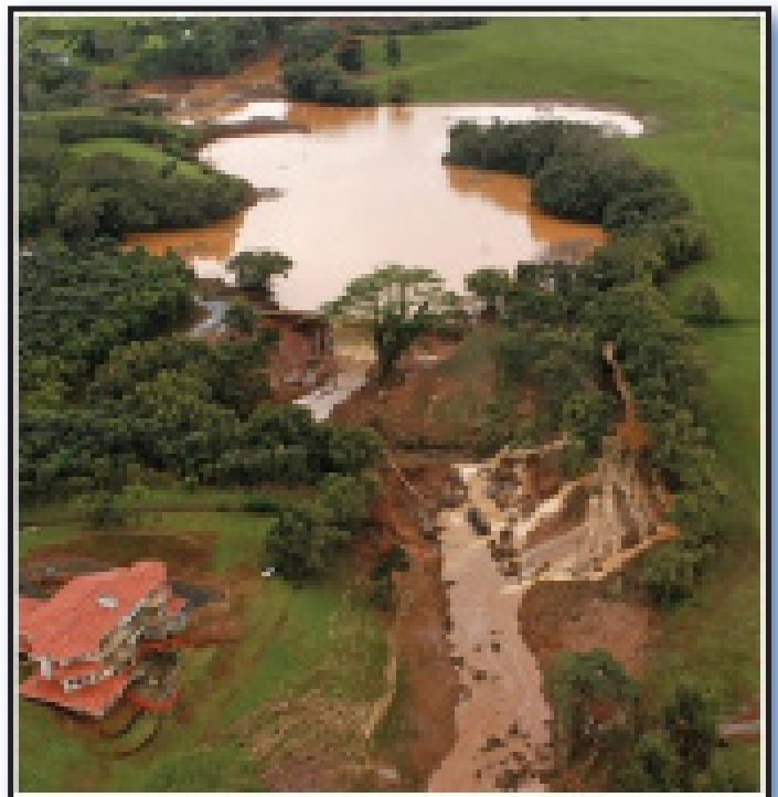
Small earthen dam embankment failure (Source: FEMA P-946)
