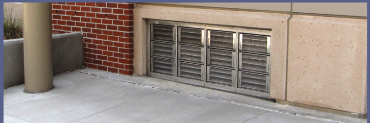
James E. Clyburn Research Center at the Medical University of South Carolina, Charleston, SC 4 x 3 multi-frame = 2,400 sq. ft. of flood protection
