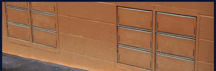
Silver Reef Hotel Casino Spa, Ferndale, WA 2 x 3 multi-frame = 1,200 sq. ft. of flood protection
