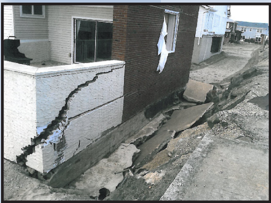
Sea Bright, New Jersey after Sandy (Photos: John Miller, PE, CFM, CSM; Associate Water Resources Engineer; Princeton Hydro, LLC)
