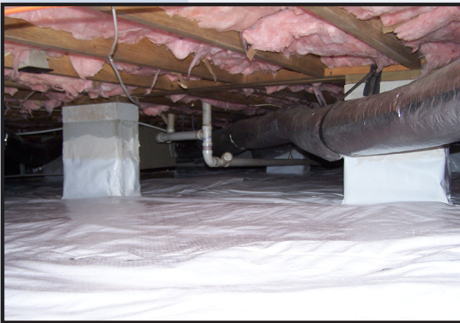
Crawl space before (top) and after (bottom)
