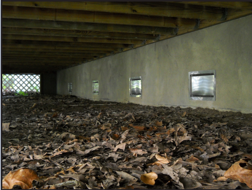
Compliant flood venting
