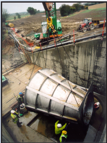
Figure 2. (above) Installation of a large vortex valve at Weedon Dam. This robust, conical-shape valve is designed to initiate a vortex during high flows, restricting the flow of water out of the device.
