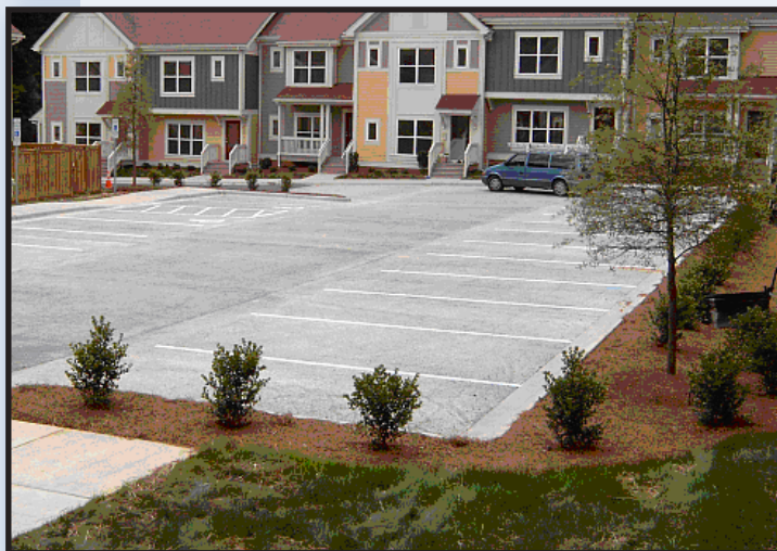
Figure 3. Completed pervious concrete and infiltration basin captures the 2-year 24-hour storm, Wilmore Walk
