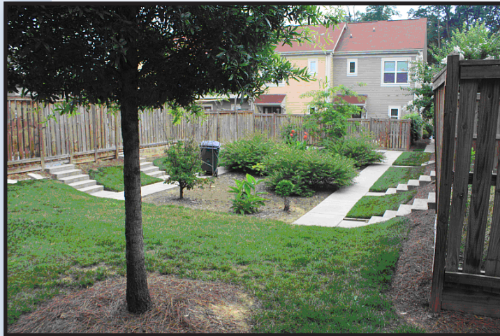
Figure 1. One of eight bio-retention cells completed at Wilmore Walk, Charlotte, NC
