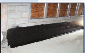
Dry floodproofing is designed so that up to a certain level, the walls are substantially impermeable to the passage of water. Structural components having the capability of resisting hydrostatic and hydrodynamic loads and effects of buoyancy must be included. The methods used can be found in FEMA *Guidance Bulletin 3-93: Non-residential Floodproofing*.
